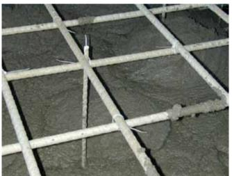
Figure 11.4: Glass FRP rebars tied with nylon zip-ties and glass FRP chairs to eliminate all corrosion (courtesy Vector Construction Group).
