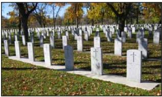
Figure 12.6: GFRP-Reinforced Cemetery Marker, Brookside Cemetery, Winnipeg, Manitoba.
