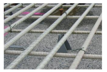
Figure 11.5: Glass FRP rebars tied with standard steel ties and using plastic chairs (courtesy Vector Construction Group).
