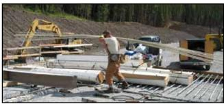
Figure 11.2: Lightweight bundles of FRP bars are easily moved on site (courtesy Vector Construction Group).
