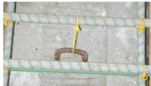
Figure 11.6: Glass FRP rebars tied down with plastic-coated steel ties (courtesy Vector Construction Group).
