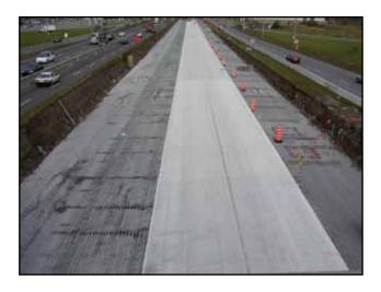
Figure 12.10: Continuous Reinforced Concrete Pavement with GFRP bars on Highway 40 East-Montreal.
