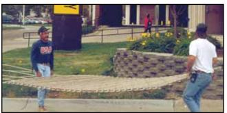
Figure 11.1: Large sections of preassembled formwork can be installed with ease (courtesy Vector Construction Group).
