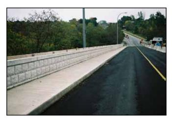
Figure 12.11: Deck Rehabilitation of Glendale Avenue Bridge.
