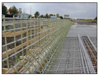
Figure 12.9: Reinforcement of the bridge deck slab and barrier walls, Val-Alain Bridge.
